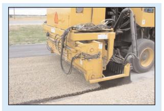
RoadArmor High Performance Chip Seal is a single pass surface treatment developed for cost-effective pavement preservation with low user delays. It is designed for high traffic roads in good condition but with minor surface distresses. A new ultrafast setting polymer modified emulsion is used with a single-sized aggregate in a continuous synchronized application.
